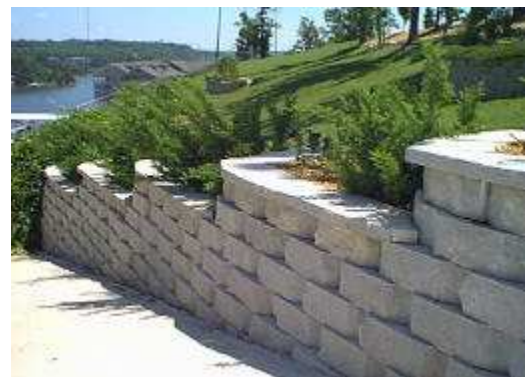
STEPPED WALL BEING TERMINATED INTO BANK
